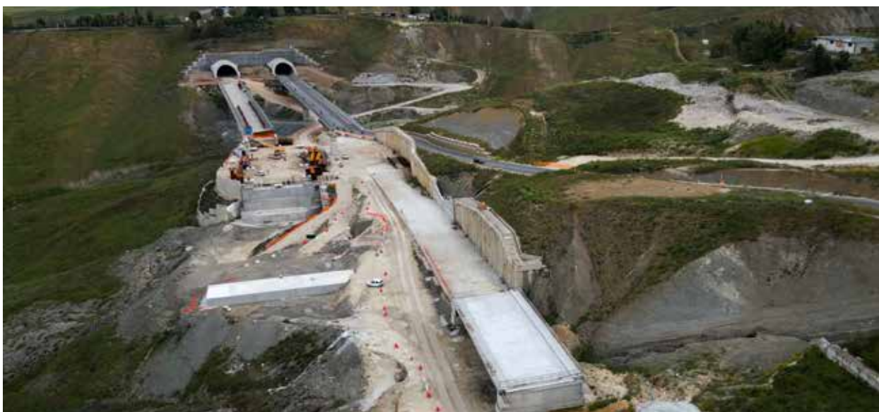
Ferroberica construction site: S.S. 640 Caltanissetta-Agrigento main road with tunnel
